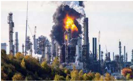
Saint John Oil Refinery
