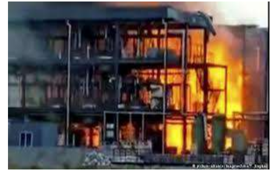
Chemical Plant Blast.
