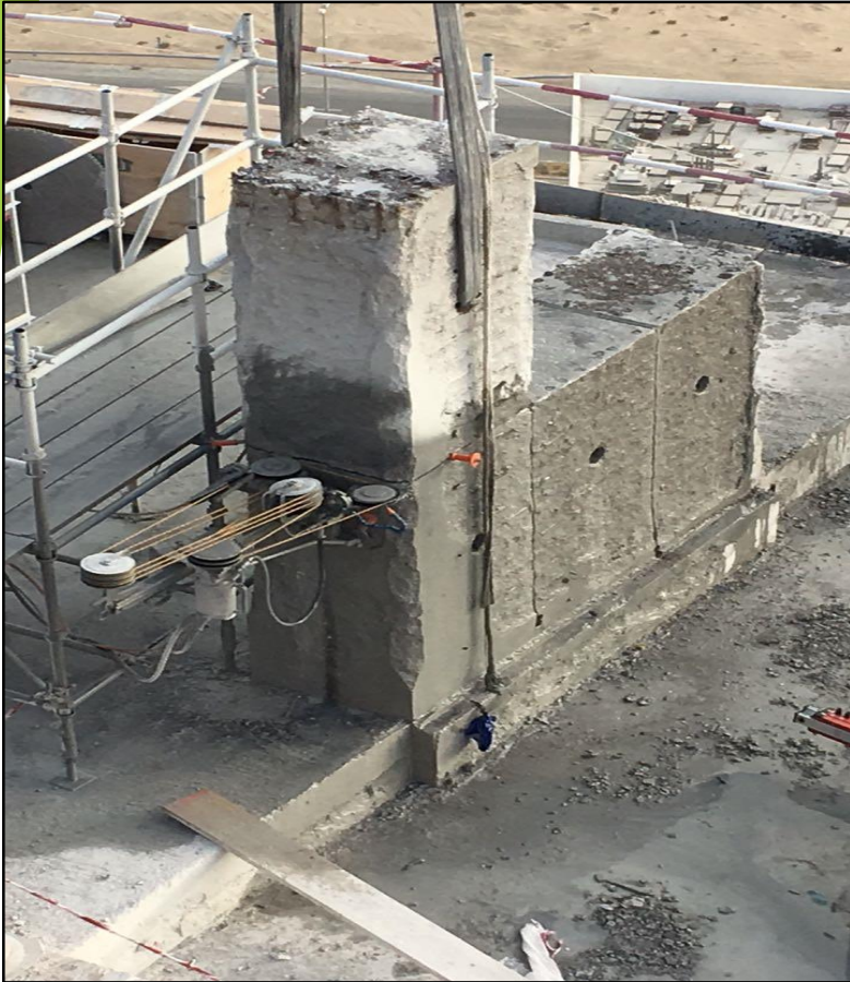
DIAMOND WIRE SAWING.
