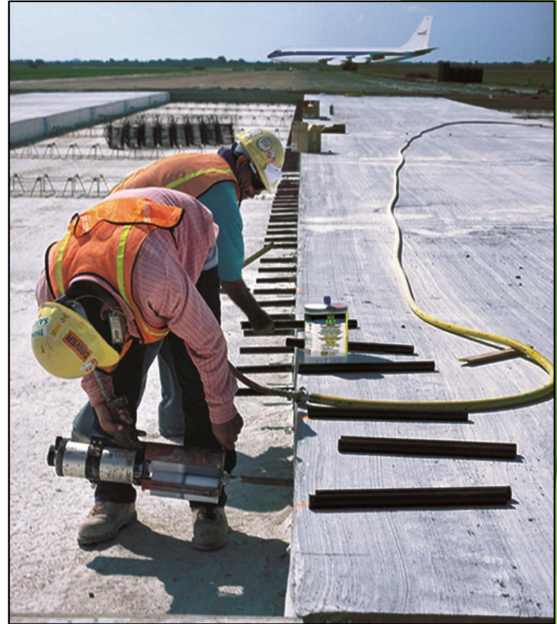
EPOXY REBAR DOWELING & ANCHORING OF RODS.
