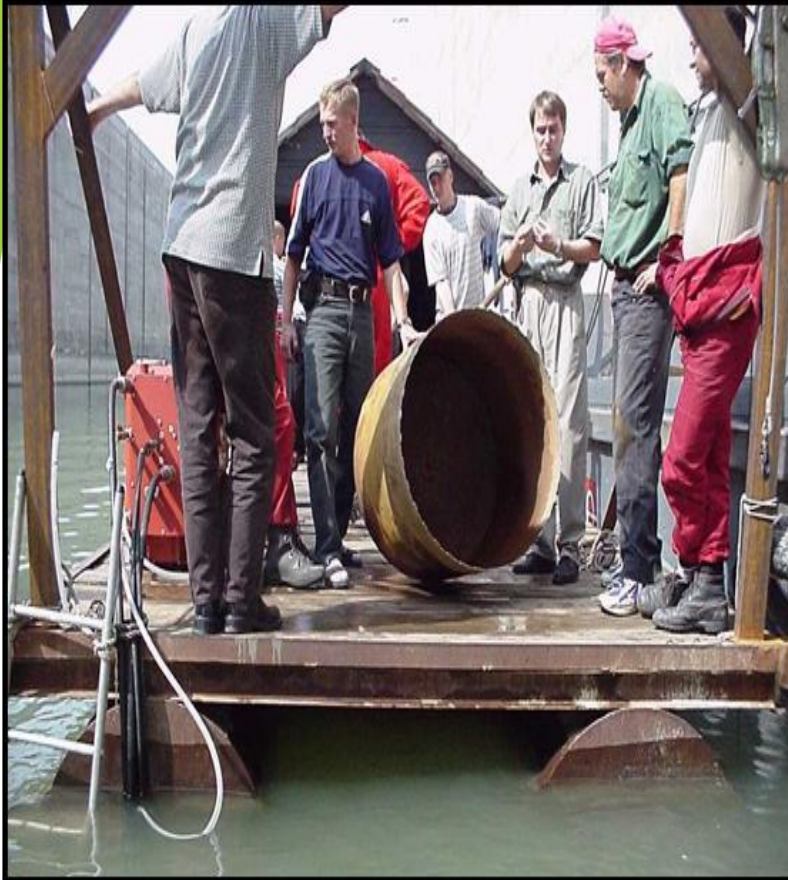
UNDER WATER DIAMOND CORE DRILLING.
