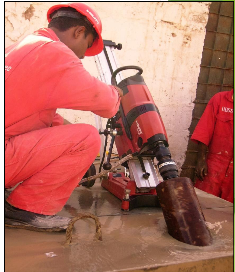
DIAMOND CORE DRILLING.
