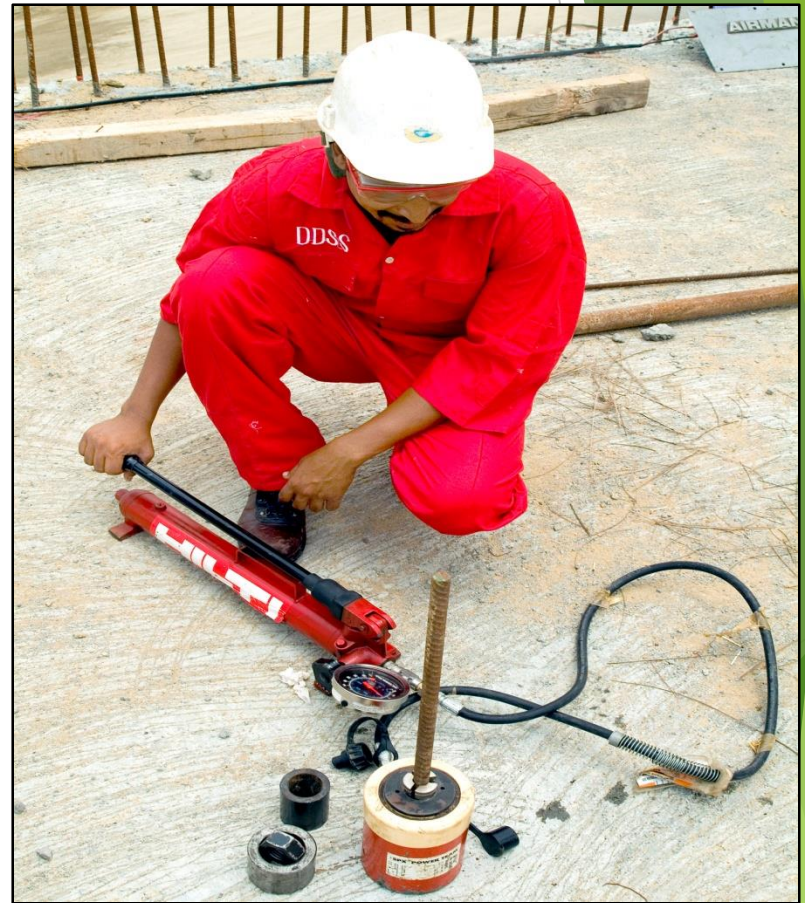
ANCHOR PULL-OUT TESTING.
